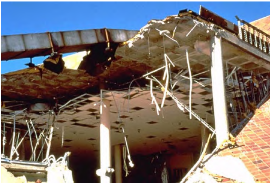
Figure 7-1 Severe damage to a department store severely shaken by the 1994 Northridge earthquake. Shear failure between the waffle slabs and columns caused the collapse of several floors. (photo courtesy of the Earthquake Engineering Research Institute.)
